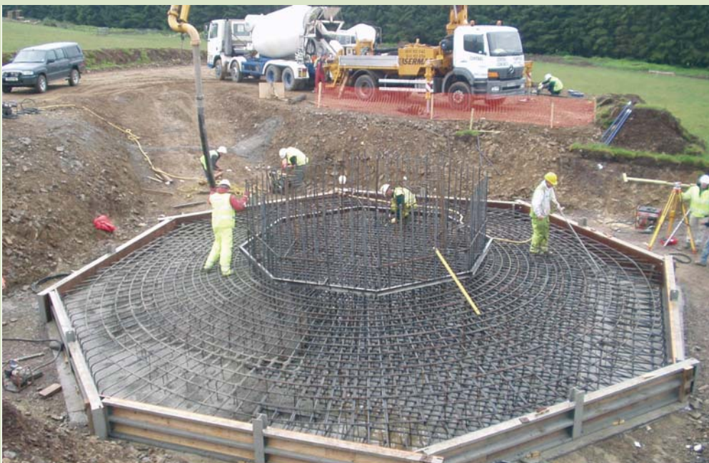
Construction of a typical wind turbine foundation
